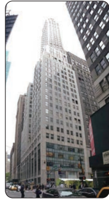
Fujitsu General Solution Centre "THE AIRSTAGE"
